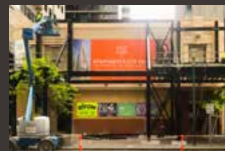
Melbourne, VIC CBD Development Site
